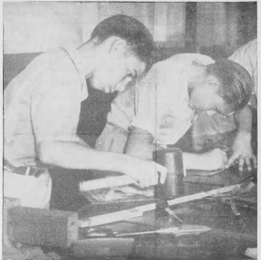
Clemente Geerman (left) uses a large mallet to hammer a double seam in a piece of sheet metal and Benito Geerman (right) marks a piece of sheet metal before cutting it. Clemente Geerman (na banda robex) ta usa un martin grandi pa e plat un pida metal y Benito Geerman (na banda drechi) ta marka un pida metal promé cu e corté.
